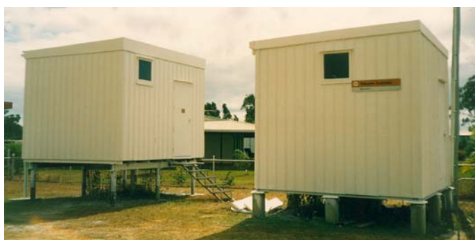
▲ Telstra Maintenance Huts.
