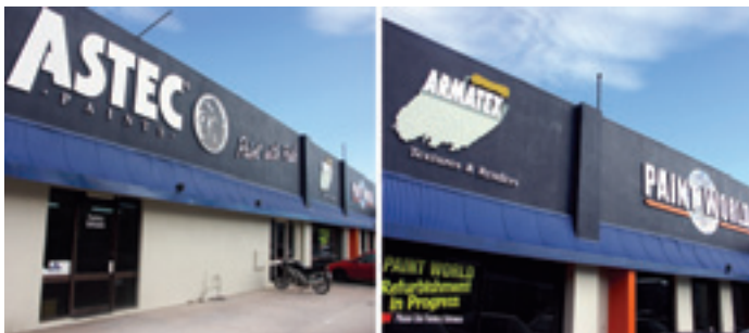
Astec Paints Renovations in progress.
